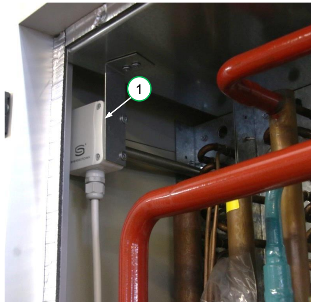
Figure 4-2. Unit Sensor
