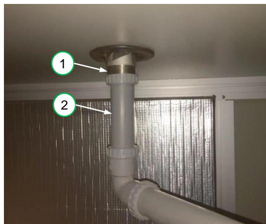
Figure 5-2. Water drain outlet
