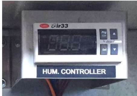
Figure 6-1. Humidistat controller
