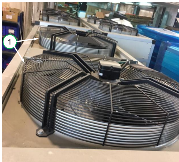
Figure 5-13. Axial blowing fans
