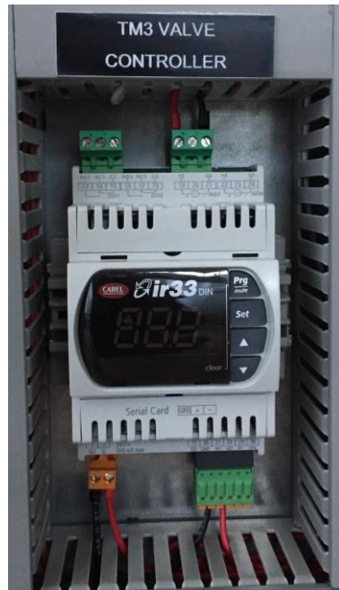
Figure 9-16. Temperature valve controller
