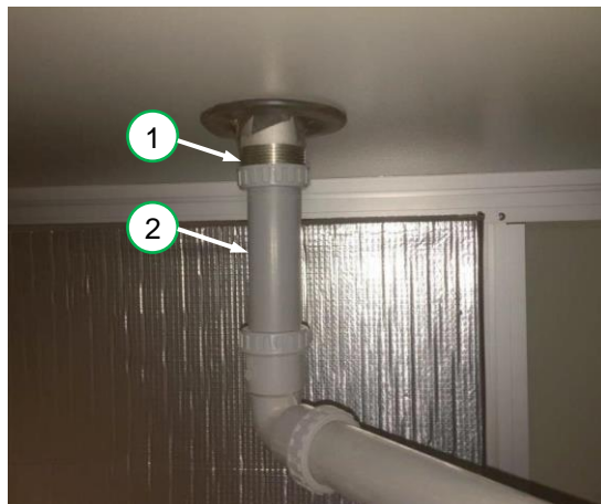
Figure 4-4. Water drain outlet
